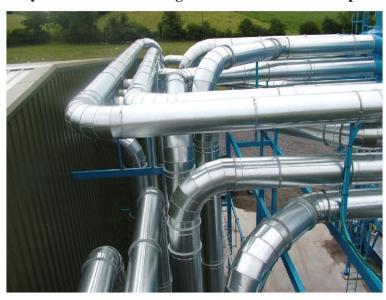
Careful design, with slow bends in place of tight ones, illustrated here with seven segments, and smooth aerodynamic branches and transitions will reduce fan power requirements continuously. Incorrect air velocity in ducting can be expensive, not only in energy costs but also in maintenance and replacement costs. If it is too high, then fan power requirement can increase markedly; but also the rate of attrition will increase. This
