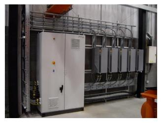
Continuous modulation of the fan speed using an inverter drive could easily save in excess of £3000 every year in this example, without even taking into account the power losses of 5% or more incurred by belt drives.
