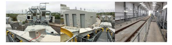
Having been unloaded the fuel pellets are then transported by a twin, air supported, belt conveying system to the main station storage silos. The six concrete slip-formed silos are fitted with a Fairport designed bottom to encourage mass flow and are also inter-connected by drag link conveyors in such a manner that the storage silos can operate on a FIFO (First In First Out) basis.
