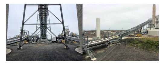
The intermediate storage silos hold the pellets prior to them being fed into 12 individual dense phase conveying systems to reach the grinding mills that will pulverise the pellets before being injected into the boiler burners. Lynemouth has three boilers and each is served by four mills each of which has four dedicated dense phase conveying systems, one of which is a hot standby.
