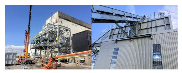
Fairport was commissioned directly by Lynemouth Power to provide a conditioning system for the finer Fly Ash. This consisted of drag link conveyors, silos, duplex discharge screw conditioners and screw conveyors to transport, store, condition and deliver the ash into skips for onward disposal. The new system is located in the same position as the existing facilities and utilises the existing structure, suitably adapted and refurbished, but with only two new holding silos.
