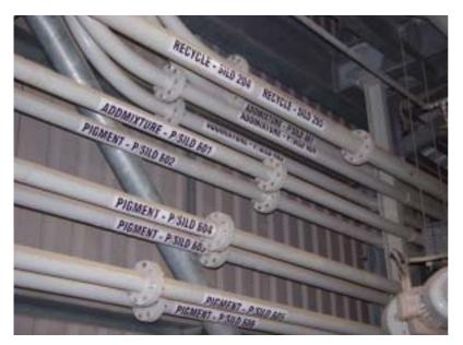
Part of the complex network of pneumatic fill pipes in the DSM plant
